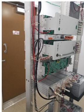
RF Site Equipment Installation
